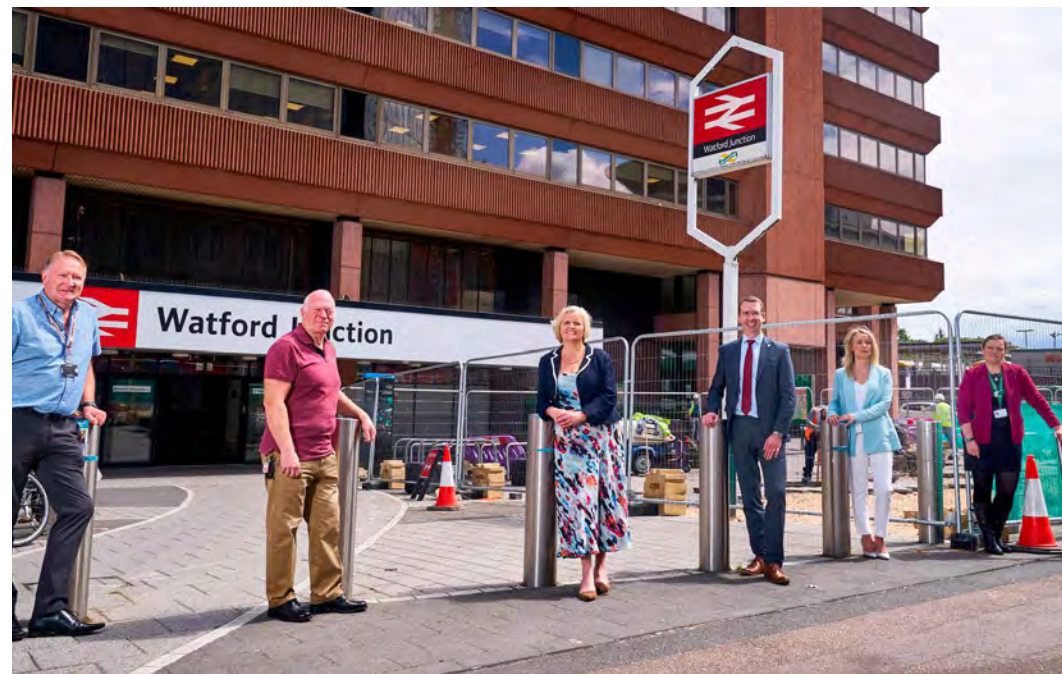
Work begins on Watford Junction forecourt
