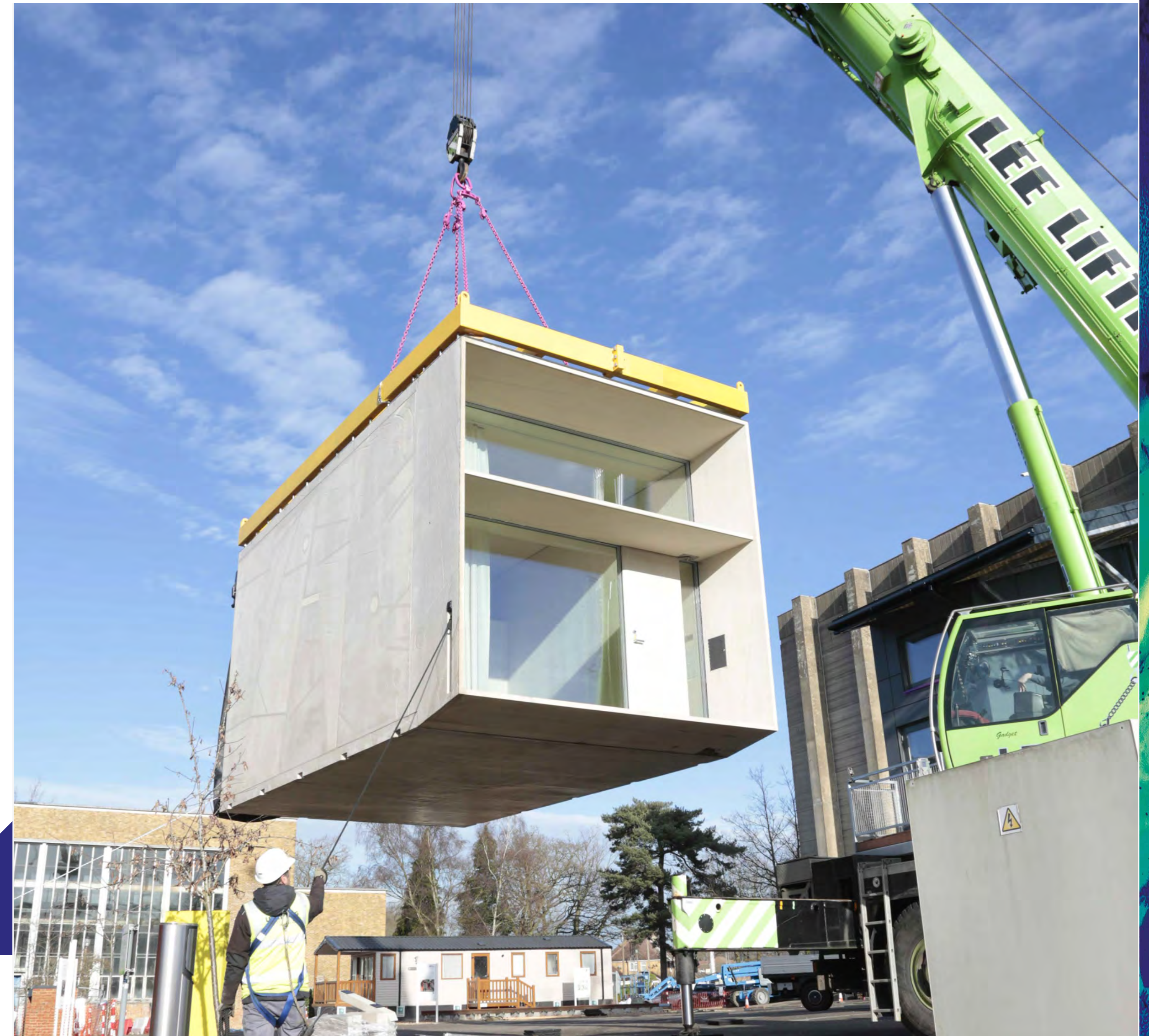
Offsite modular construction
