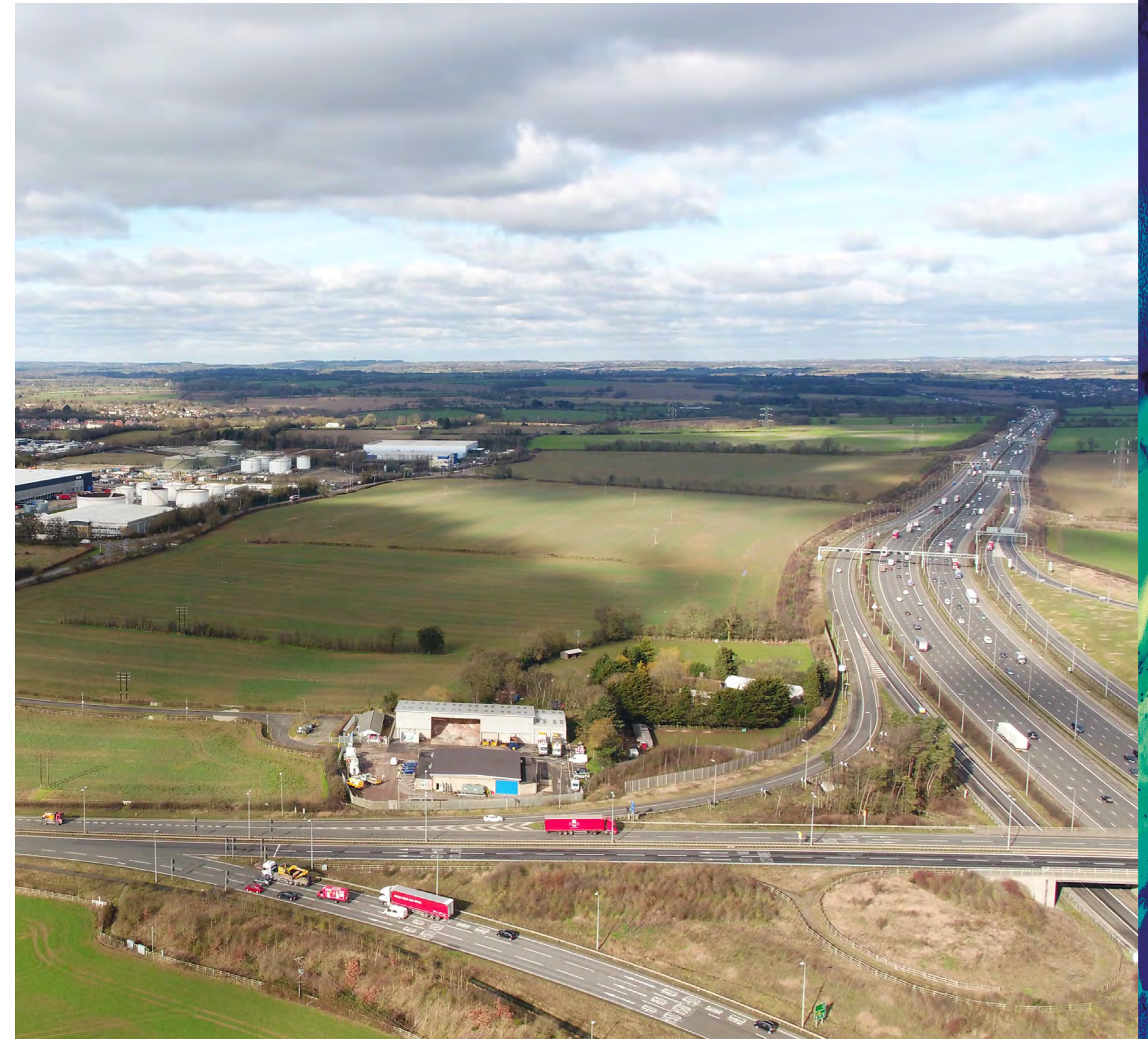
£6m M1 Junction 8 design project underway, with £3m Local Growth Fund investment from Hertfordshire LEP matched with £3m from The Crown Estate.
