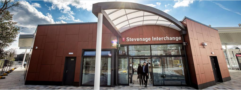
Stevenage town centre regeneration
